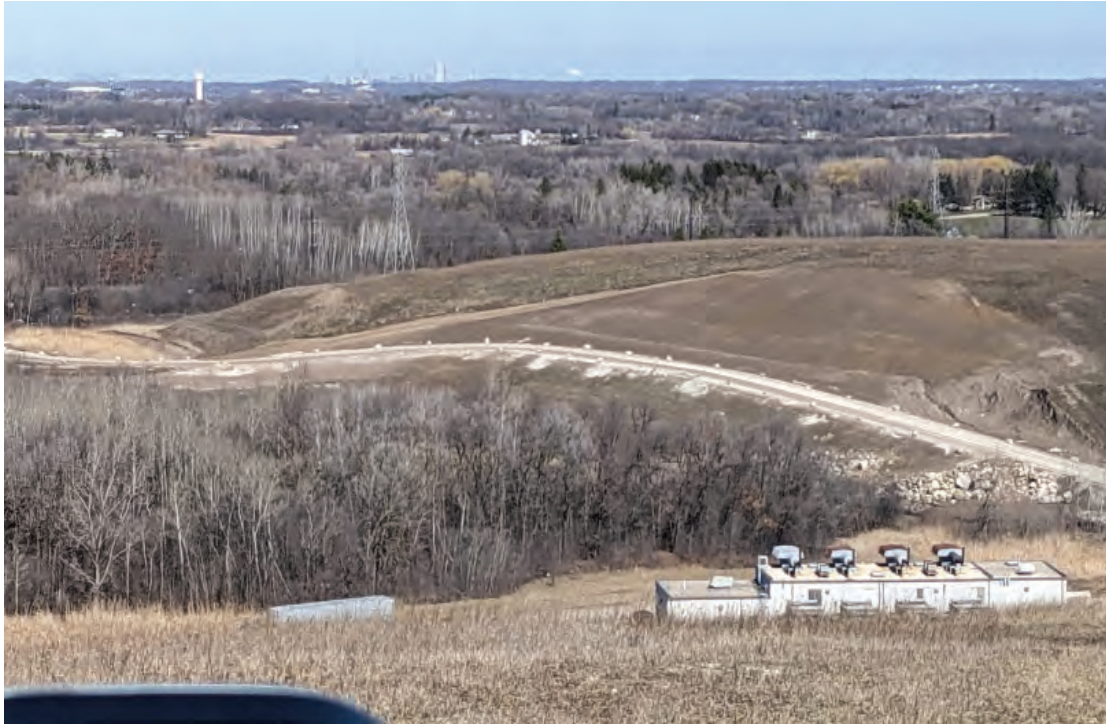
Stock pile and access road to North Expansion West
