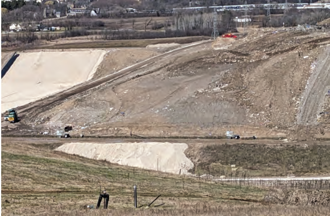
South slope of North Expansion West, fully covered in intermediate cover
