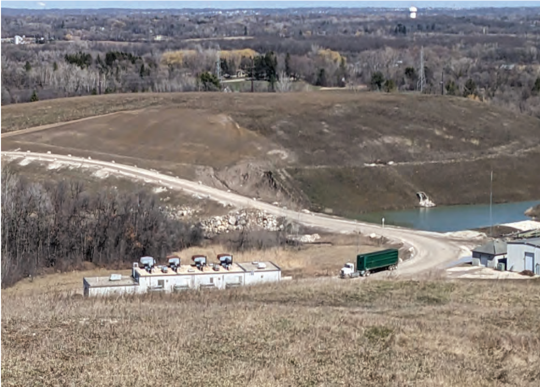
Long access road run from scale house, past gas plant to stockpile before reaching North Expansion West
